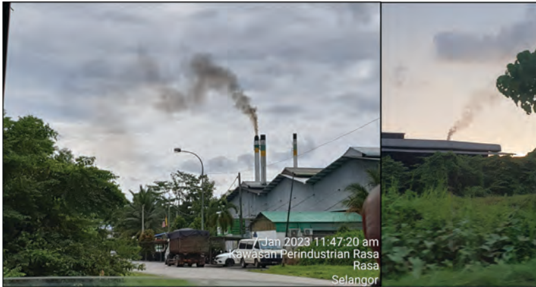
Figure 4.4: Clear violation of air pollution regulations, Rasa (Selangor), 7 January 2023; Telok Panglima Garang (Selangor), 7 November 2023
